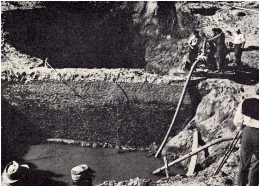
Fig. 5. Excavation of the long wall which was located with the proton magnetometer. A Roman wall was constructed on the Greek wall which appears just above the water line. [Photograph by J. Delmege, University Museum.]
